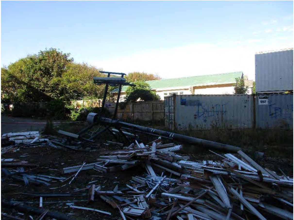
Photograph 7: Area formerly occupied by Marae building, now temporarily containing demolition materials.
