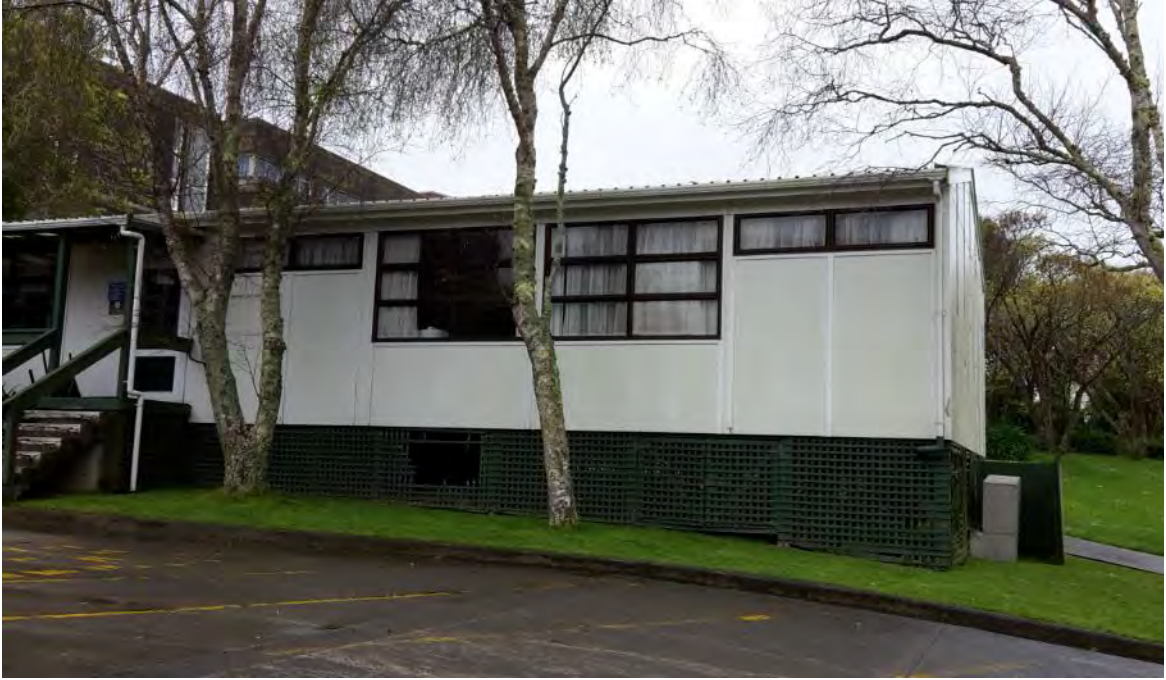
Photograph 3: A typical pre-fabricated building.
