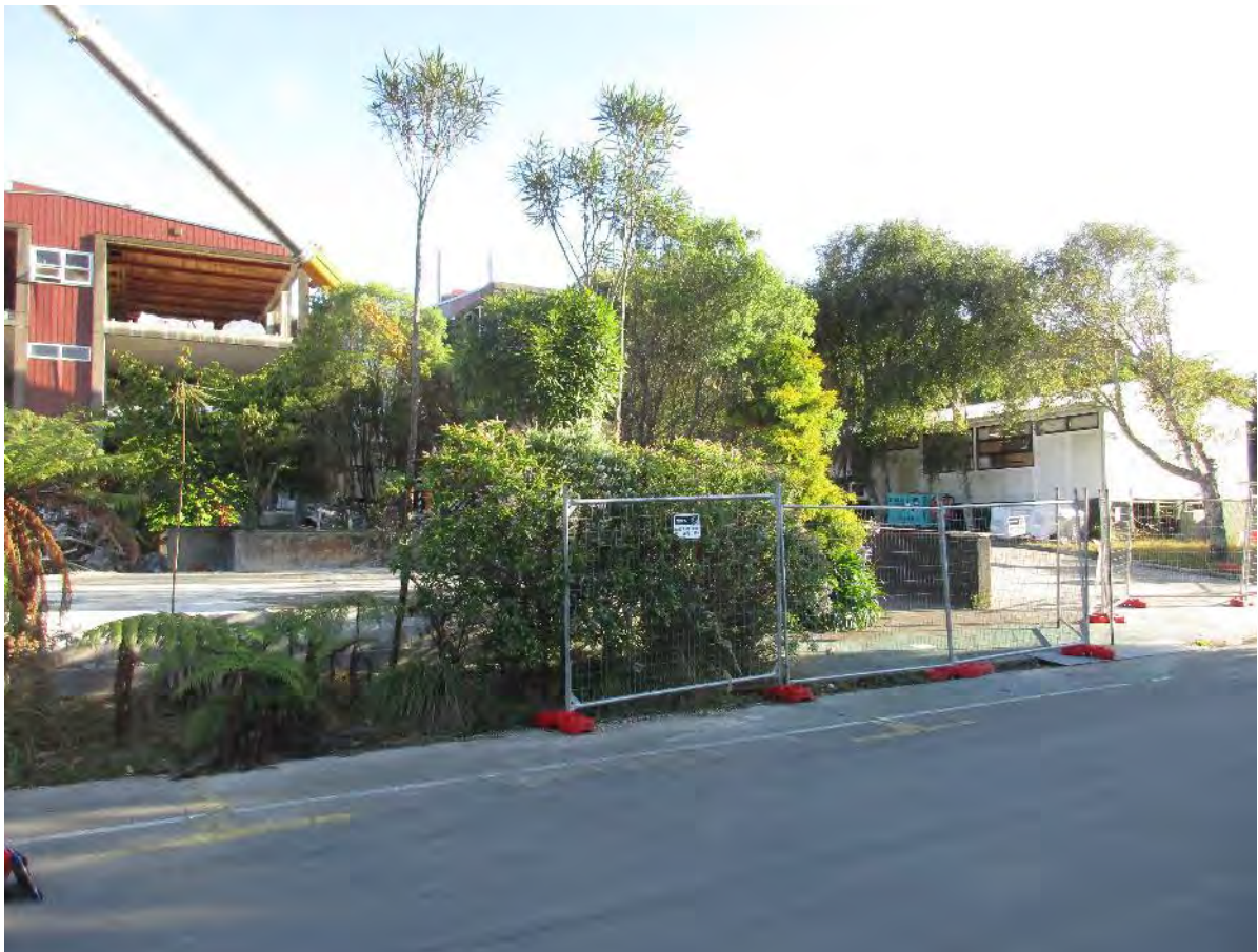
Photograph 6: View of footprint of Mackie Gym building following removal.
