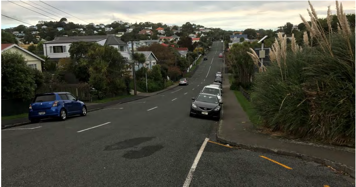
Photograph 1: Available sight distance from main entrance (east) looking south (Donald Street)
