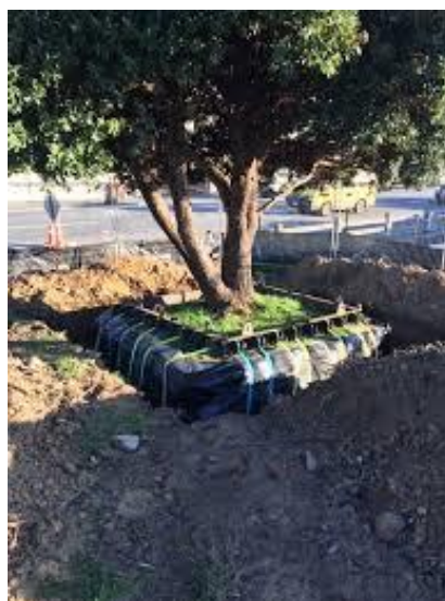
Photograph 1. Tree framed and ready for lifting.
