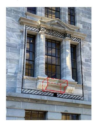
The SPA Design Statement Figure 33 showing the 3-part window where the link bridge will enter PH. The red line indicates where the stone will be cut away. The black line shows where the bridge link will contact the PH façade.
