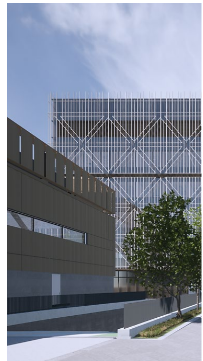
Figure 3.13 Detail of lattice with diamond motif and horizontal datum at Level 4.
