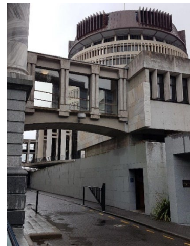
Figure 3.19 Existing link bridge, viewed from the west.
