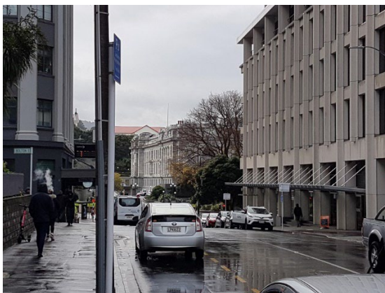
Figure 1.7 Looking south along The Terrace – the western facade of Parliament House framing the edge of Museum Street (not in view).
