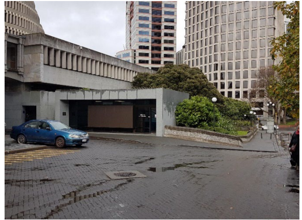
Figure 1.4 Existing Mail Screening Building (circa 2004) at the rear of the podium.
