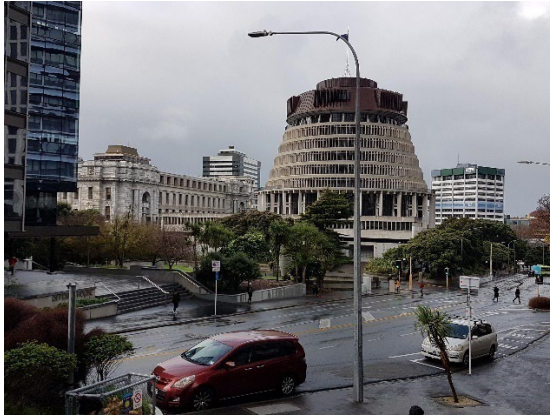
Figure 1.9 View across Bowen Street showing the Beehive as a prominent element with the Sculpture Park (at left) in the foreground.
