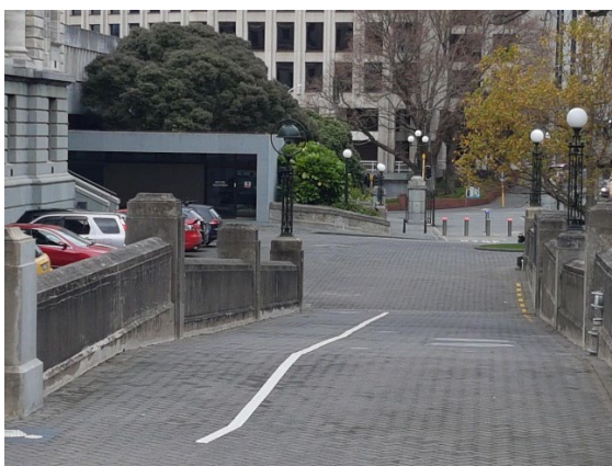
Figure 1.13 Museum Street looking south from behind Parliament House. Horizontal and vertical changes in the alignment of kerbs are evident.
