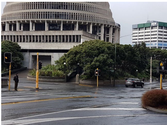
Figure 1.5 Existing Press Gallery viewed from across Bowen Street with vehicle entry in view.
