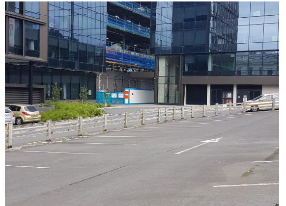
Figure 1.18 View over existing carparking area towards the north end of Bowen State Building and the east facade of Charles Ferguson Tower.
