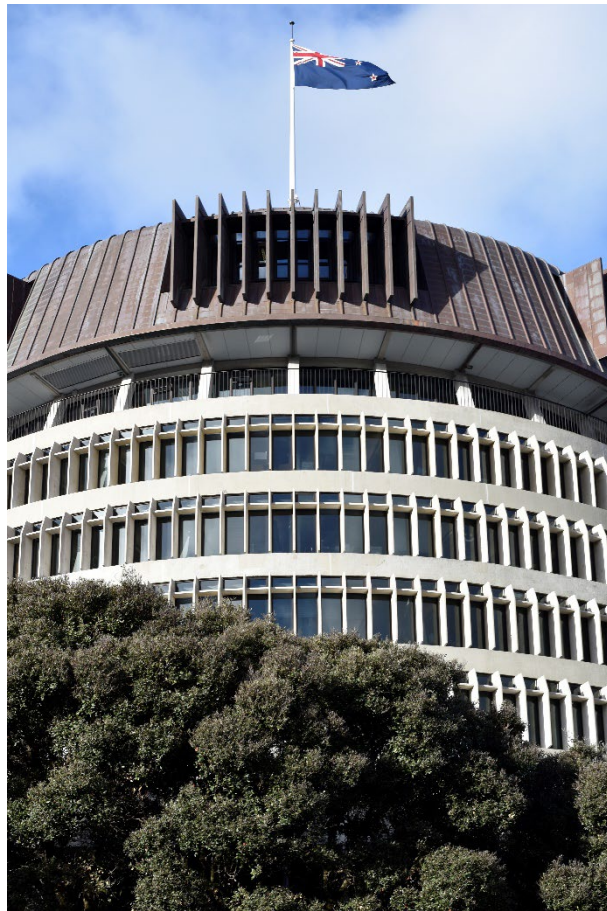
fig. 1 the executive wing. 20 may 2021 archifact – architecture & conservation ltd
