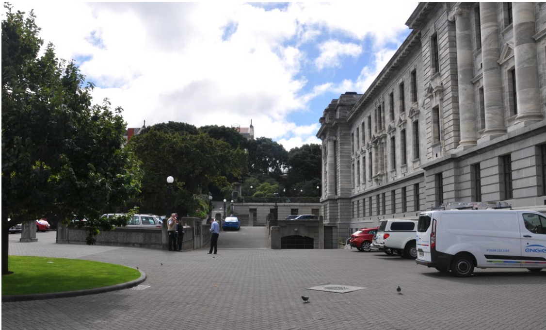
Figure 1 the existing ground condition immediately west of PH showing the at grade car parking against PH, the existing “slot” and the variation in ground level expressed by the ramp
