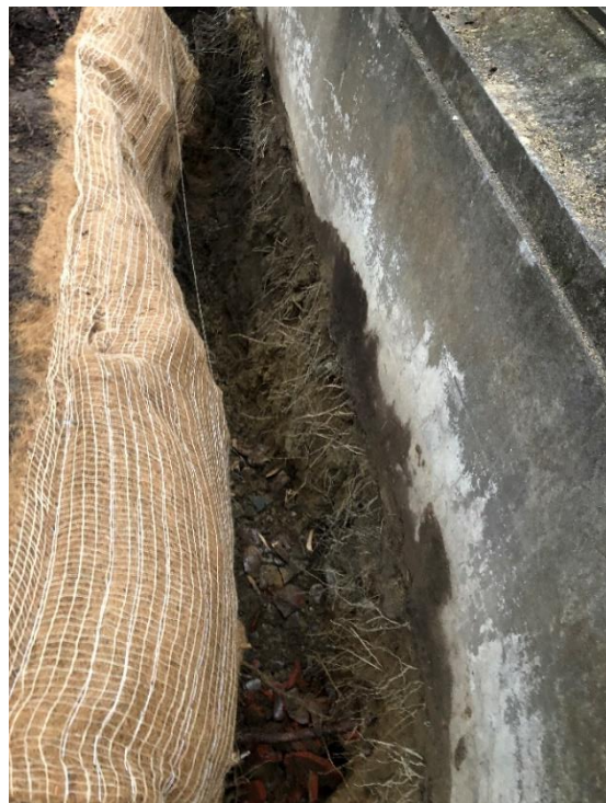
Photographs 3 and 4. Roots covered with coconut matting at the end of day 1.
