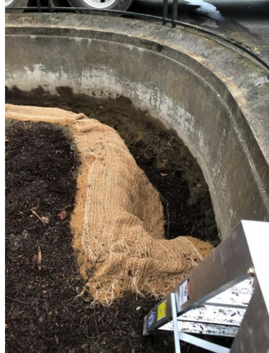
Photographs 1 and 2. Exposed roots protected during air excavation
