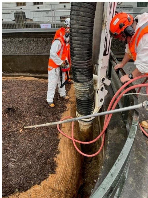
Photographs 3 and 4. The excavation work in progress.
