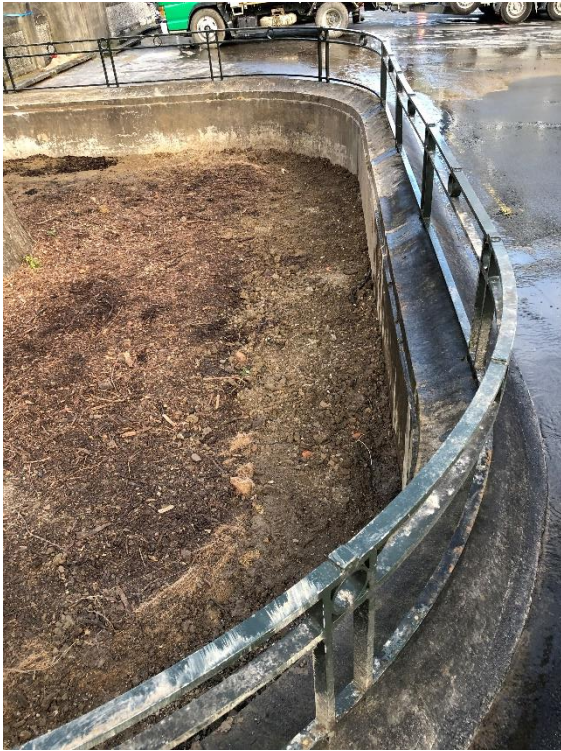
Photographs 12 and 13. Back filled excavations on the Western and Southern sides respectively.
