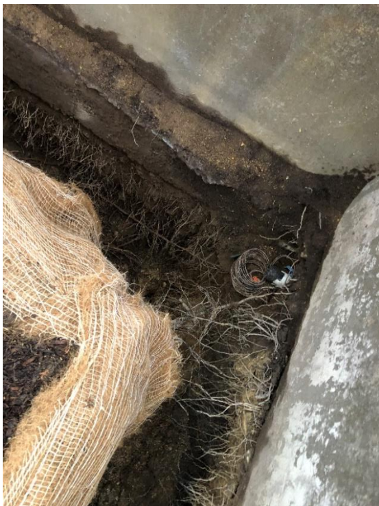
Photographs 3 and 4. Roots covered with coconut matting at the end of day 1.
