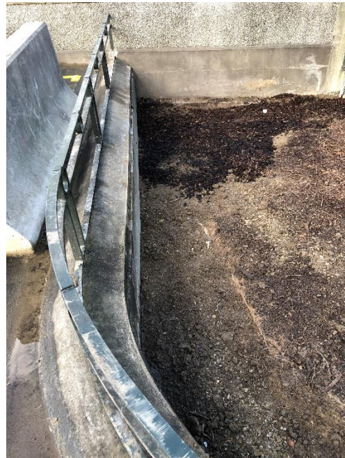
Photographs 10 and 11. Back filled excavations on the Eastern and Northern sides respectively.
