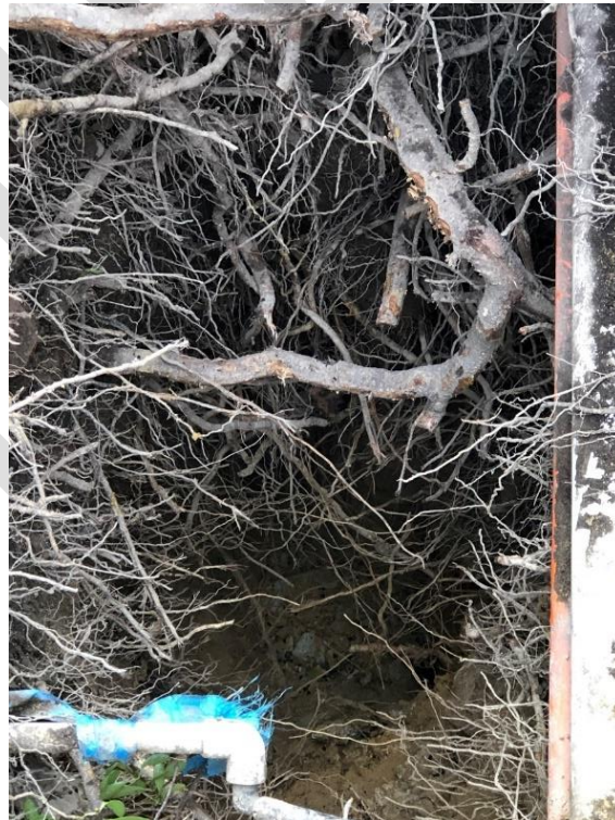
Photograph 1. Southeast corner of root zone depth to 1.8m
