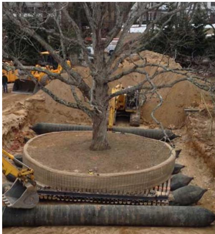
Photograph 4. Example of Large Tree Relocation Utilising Pipes and Air Bags 2
