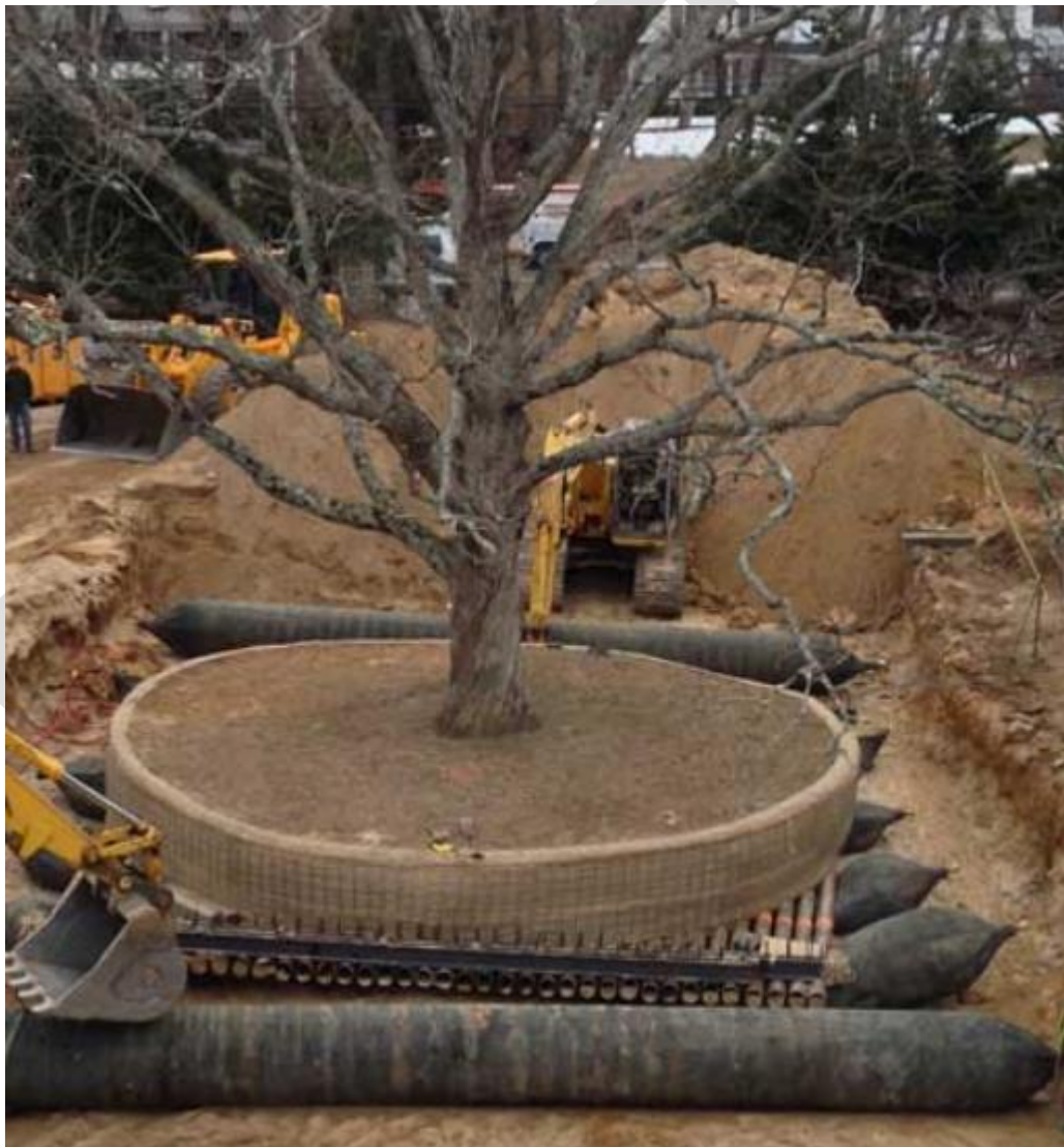
Photograph 4. Example of Large Tree Relocation Utilising Pipes and Air Bags
