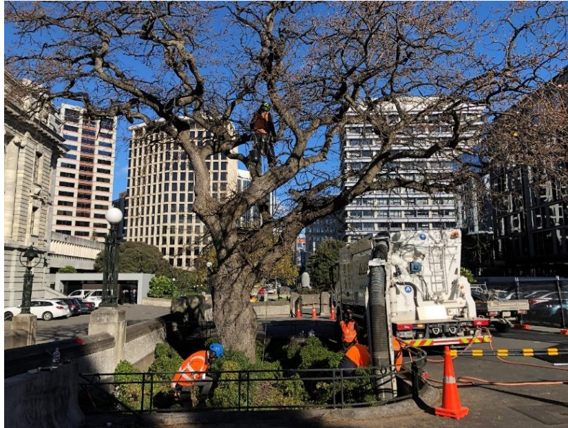
Photograph 1. Air excavation with an air vac.
