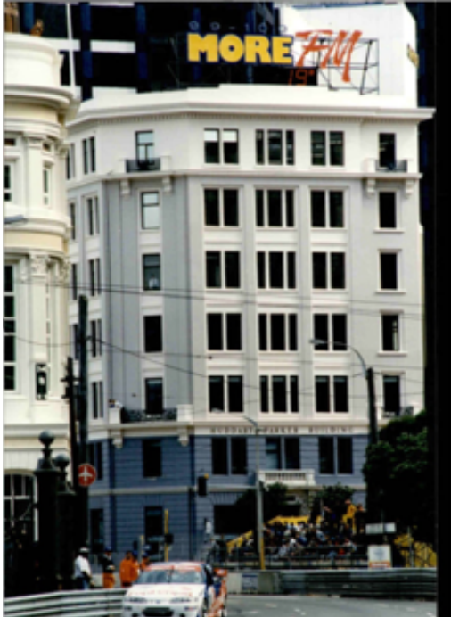
Figure 3: 'rooftop signs on Huddart Parker Building - first erected in 1963 and removed during earthquake strengthening work which commenced in 2012
