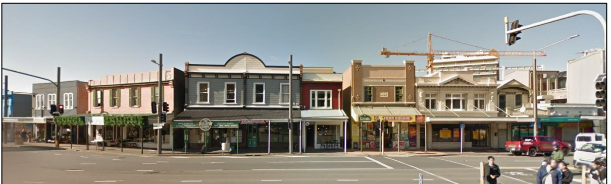
Group of early commercial buildings at junction of Adelaide Road and Riddiford Street (Google Maps).
