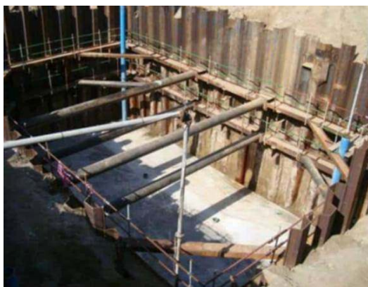
Figure 3: Propped support of earthworks option
