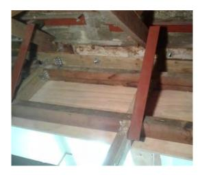
The works meet the legal URM parapet and façade securing requirements but did not address the seismic capacity of the primary structure. The strengthening also did not address the out-of-plane capacity of URM walls on connection of URM walls at first floor and ground levels.
