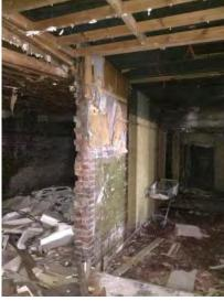
To remedy the timber decay issue, affected members would need to be removed and replaced including timber piled foundations. This would be a very involved process, propping of the facade would likely be required to allow for the replacement of damaged timber structure in the first floor.
