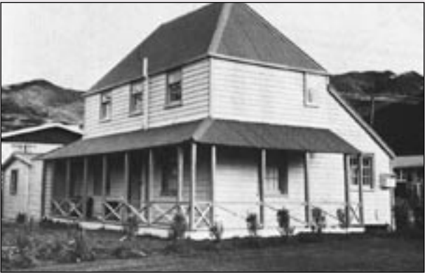
Daisy Hill Farm House from the northeast. (New Zealand Historic Places Trust)
