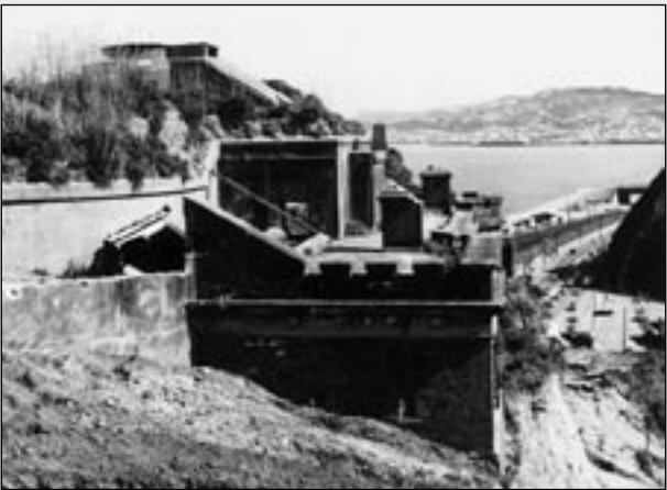
Fort Kelburne just before demolition in 1963. (25158½, ATL)
