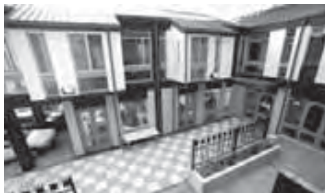
The courtyard outside Downtown Community Ministry's groundfloor offices in Lukes Lane.
