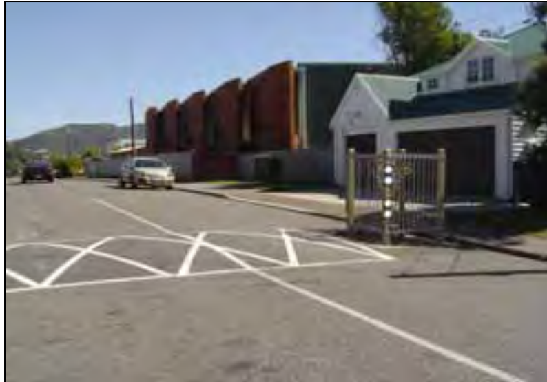
Photograph 5.3.1 - Example of a speed hump with tree and tree protector
