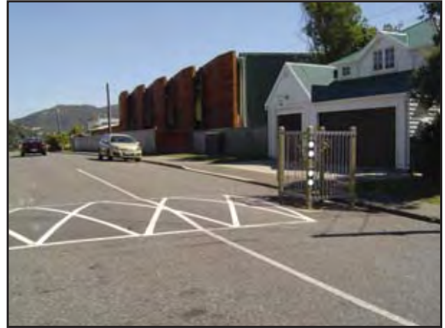
Speed humps are a proven method of reducing speed on residential streets.
