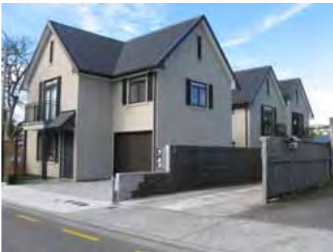
Example of a new medium density infill development within close proximity of the Johnsonville Commercial Centre
