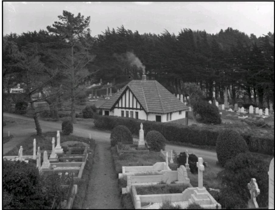
Figure 9 - The Mess and Toolshed in 1927 soon after its completion (and before additions). (ATL G247521 1/1)
