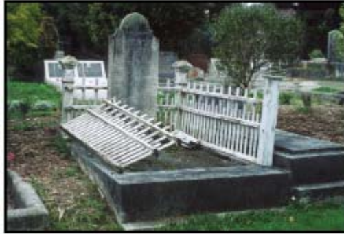
Figures 7 and 8. On left a collapsed timber fence, and on right a tilting monument, broken grave wall and components of wrought iron railing missing.
