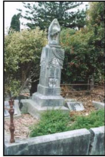
Figures 7 and 8. On left a collapsed timber fence, and on right a tilting monument, broken grave wall and components of wrought iron railing missing.
