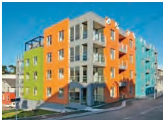
New apartment building on corner of Hanson Street and Drummond Street (2008)
