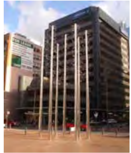
Optimisation House(right) as seen from Post Office Square
