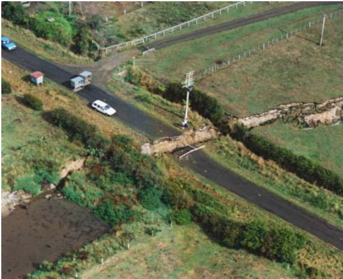
Figure 3 The 1987 fault rupture of the Edgcumbe fault at McCracken Road (Photo: D.L. Homer, GNS GNS10115-37).
