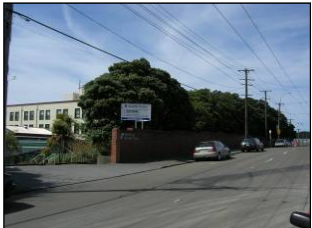
Wakefield Hospital – Rintoul Street frontage
