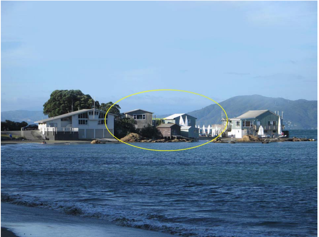
Figure 1 Existing Building View
