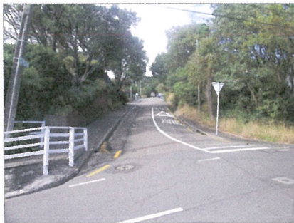
Weld Street/Cecil Road intersection.
