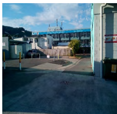
Viewed from Carpark end
