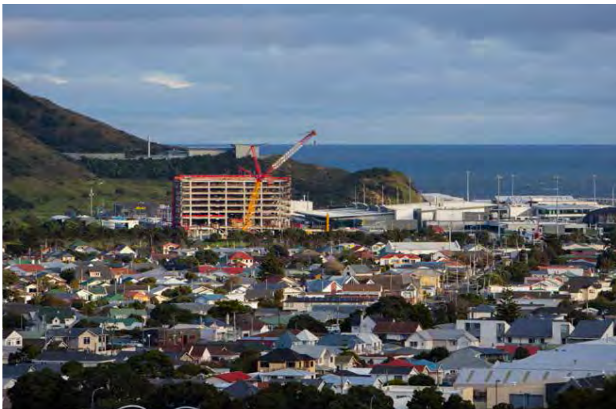
New airport hotel and car park
