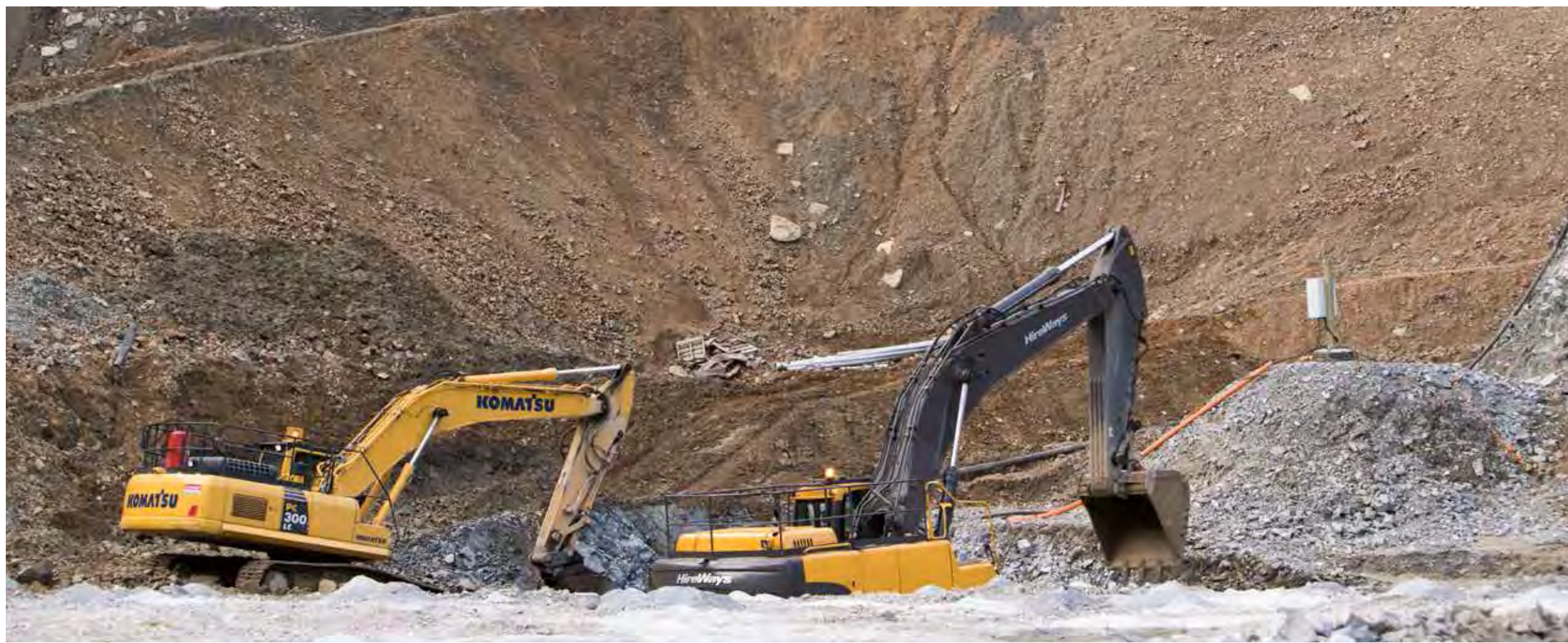
Excavation on the north face of Kiwi Point Quarry
