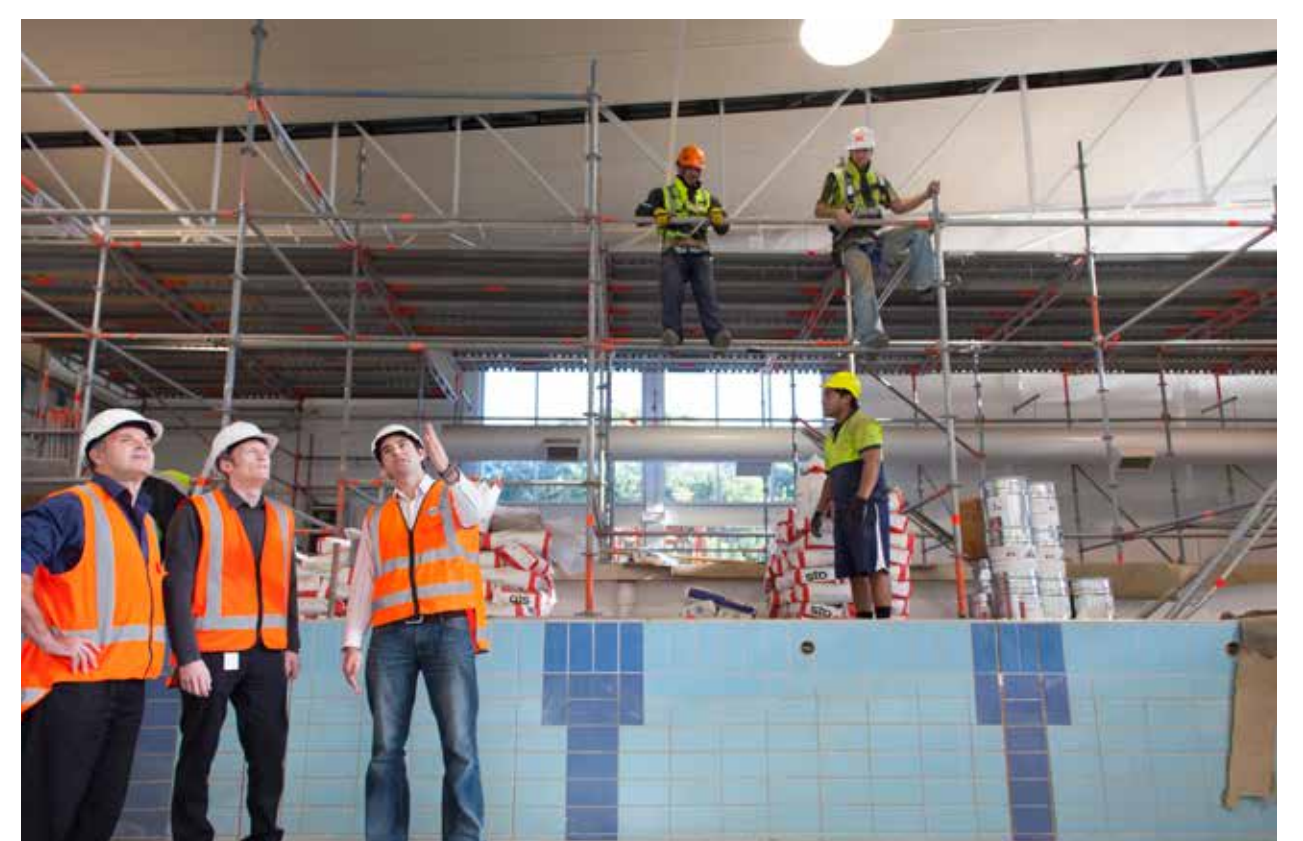
Tawa Pool Construction
