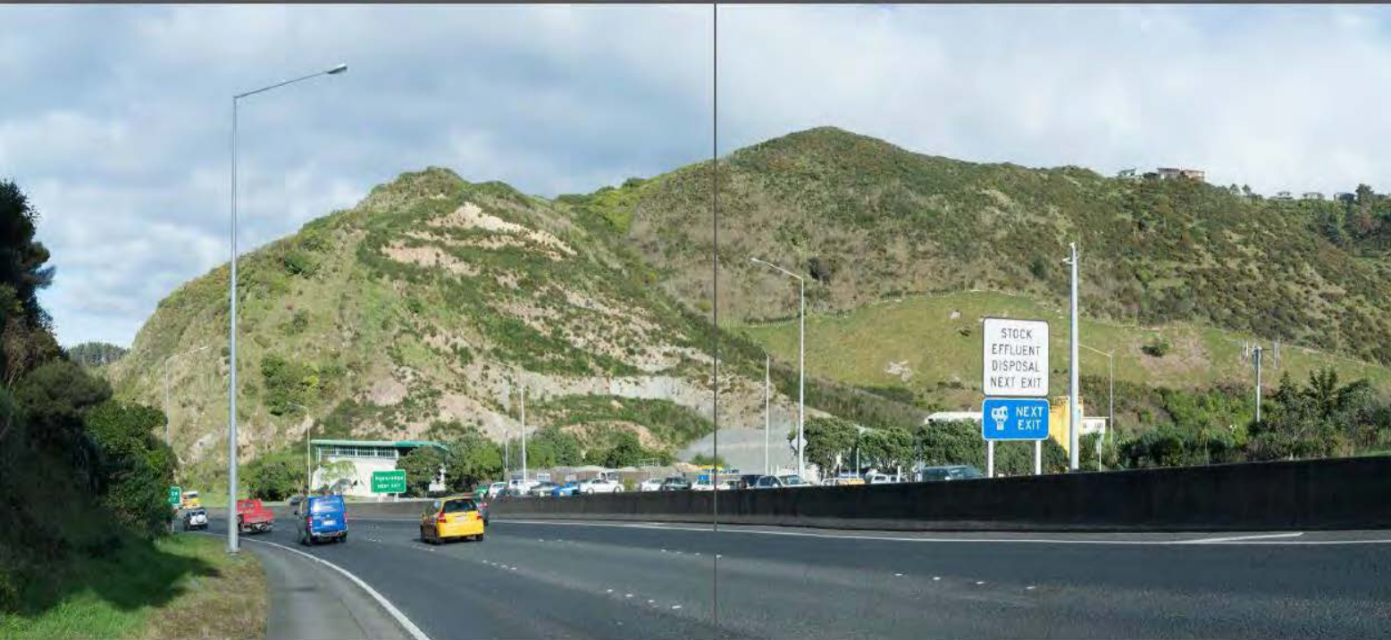
SH 1 Existing view
