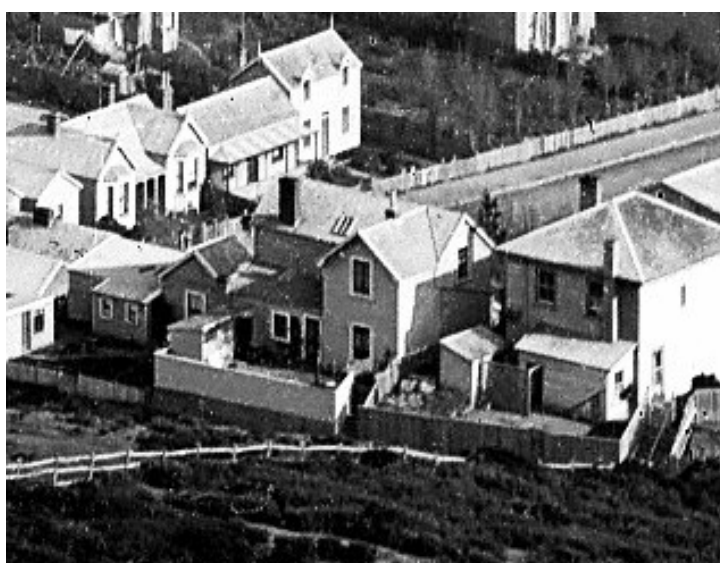
No.28 (left) pictured from the rear in 1884. At this stage the entire roof of the two storey portion was clad in shingles and like no.26 next door (right) it had a lean-to at the rear and an outbuilding. (BB-2235-1-1-G, Alexander Turnbull Library)
