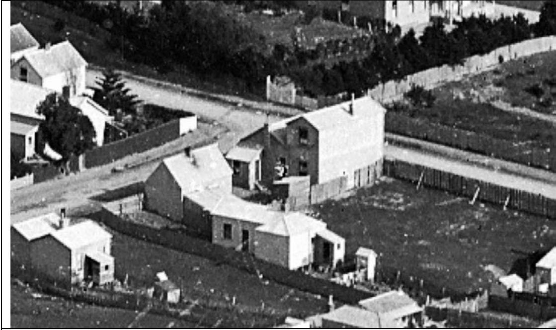
The shop and dwelling, 1884, with the bakehouse behind. (ATL, BB-2235-1-1-G)
