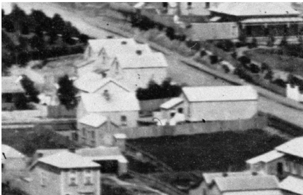
This detail from a larger image was taken in 1878, the year the shop and bakehouse (shown here enclosed by a fence) were built. (PA1-o-041-1, ATL)
