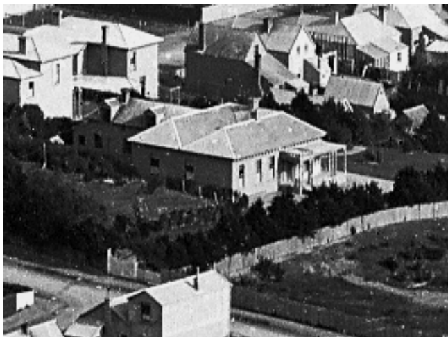
The Carroll's house, 1884. Note the servants' wing to the left and the verandah ending halfway around the north elevation at the entrance portico. (BB-2235-1-1-G, Alexander Turnbull Library)
