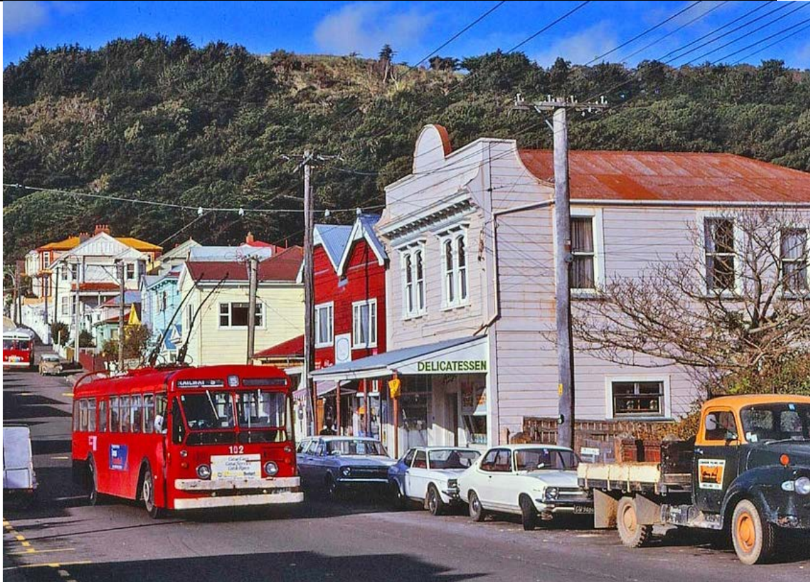
The building in 1980, before the balcony was added to the first floor. (Leroy Demory)
