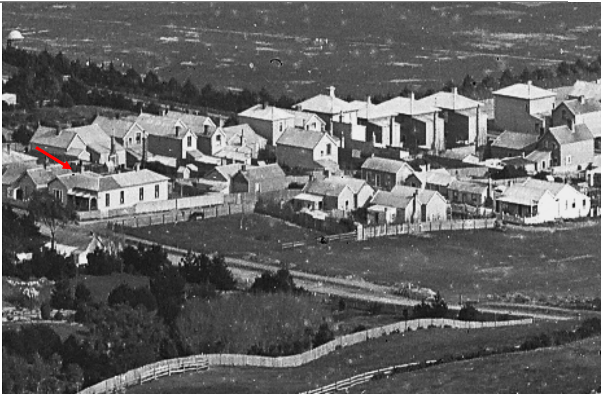
134 Brougham Street (arrowed) in 1884, with the corrugated iron clad extension to the rear. The recently formed Moir Street runs alongside the house. (BB-2235-1-1-G, Alexander Turnbull Library)
