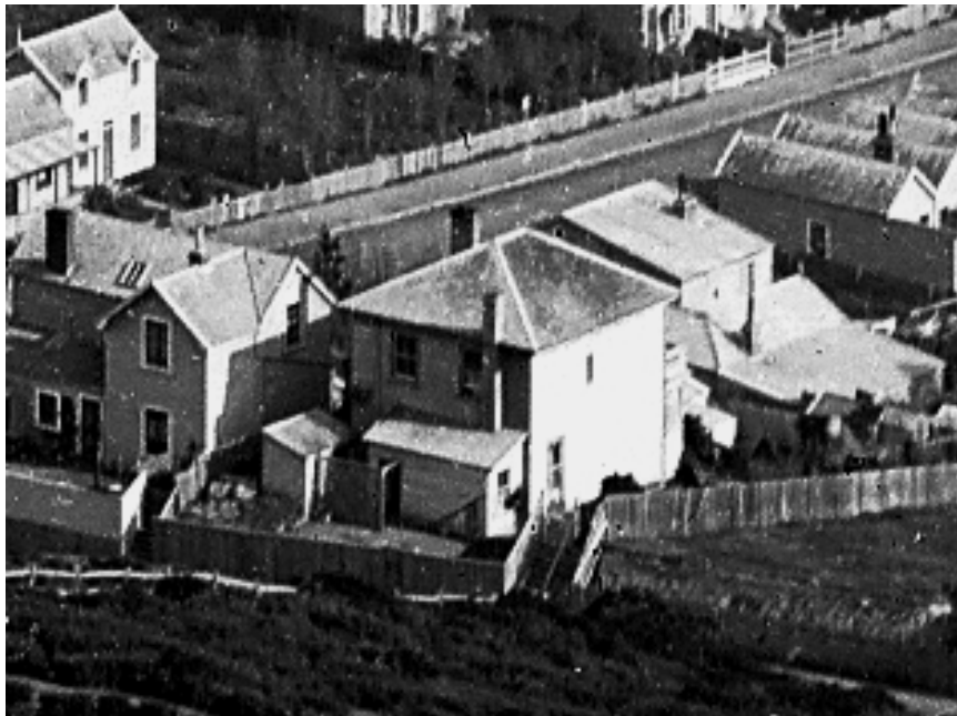
26 Austin Street during the Costalls' occupation. Note the shingle roof, lean-to and shed at the rear of the house. (BB-2235-1-1-G, Alexander Turnbull Library)
