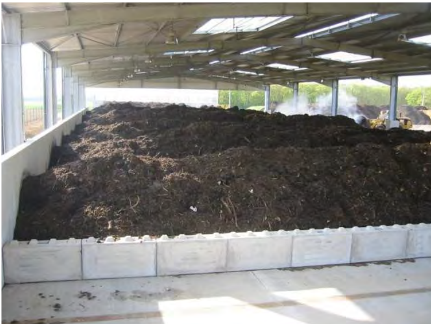
Figure 9: Example of a Traditional Composting Bund
