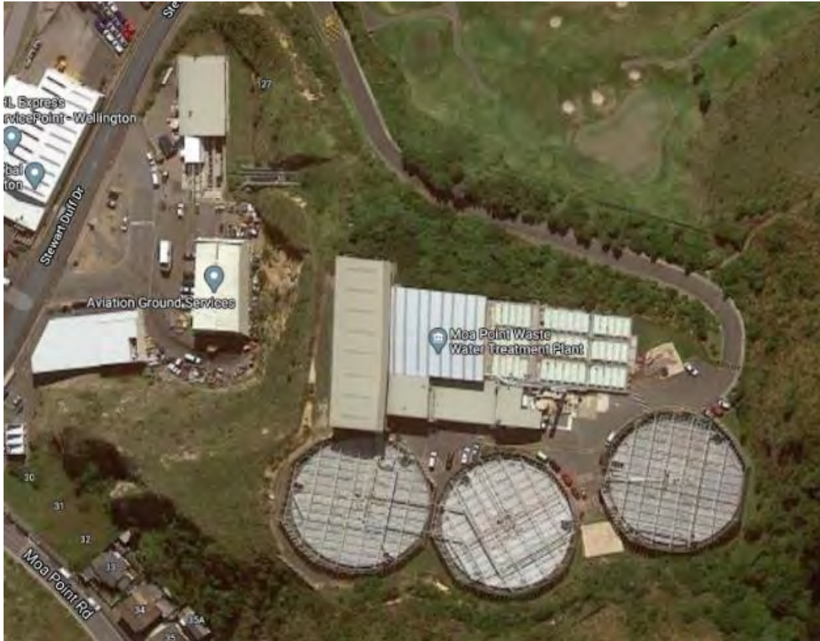
Figure 6-7: Pumping Station Substations 1 & 2 2000kVA and Moa Point Substation 3 & 4 2000kVA
